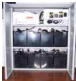
Backup batteries power can be checked automatically with their internal alarm system. When their alarm status wants to be monitored over PC, ANC series present best solution thanks to its modbus communication.
