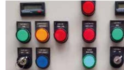
Instead of using separate alarm indicator lights, using signal modules gives you opportunity to save space and installation time with monitoring all signals in same window.
