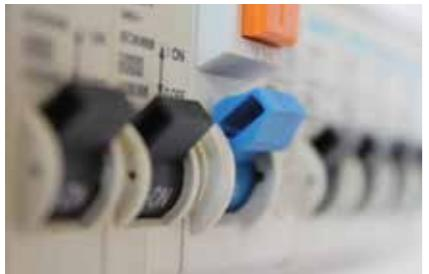
Detect a fault condition and interrupt current flow with adjustable time delay. After the fault is gone, unlike a circuit breaker, smart MCB turns its normal position automatically.
